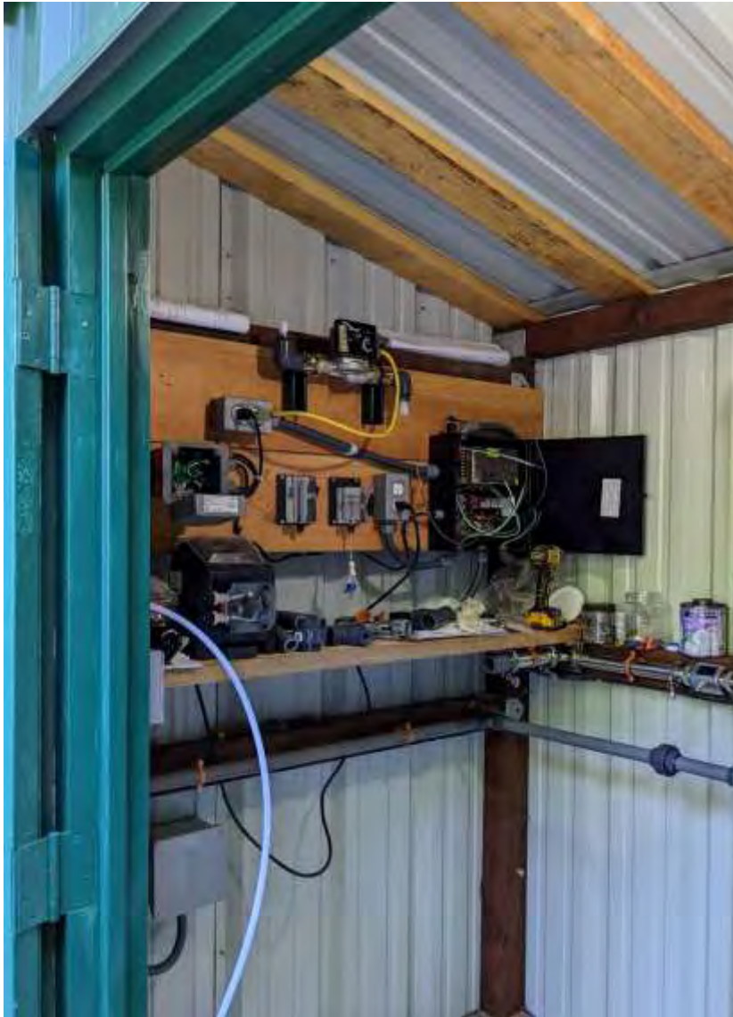
Task 3-2 – Well 2 Activation: Ozonator and filtration equipment installation in progress:
