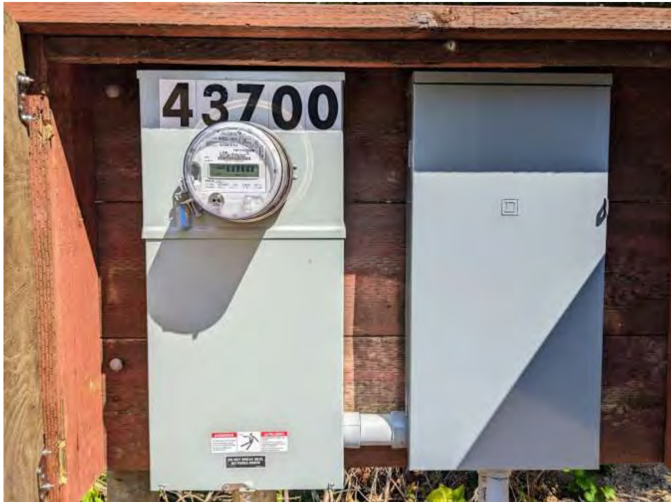
Task 3-2 – Well 2 Activation: Electrical meter base installed:
